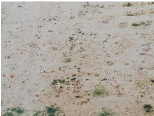
Fig 7. Algae grow inside the solar crop dryer and uneven concrete floor
