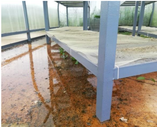
Fig 6. Insects and algae grow inside the solar crop dryer
