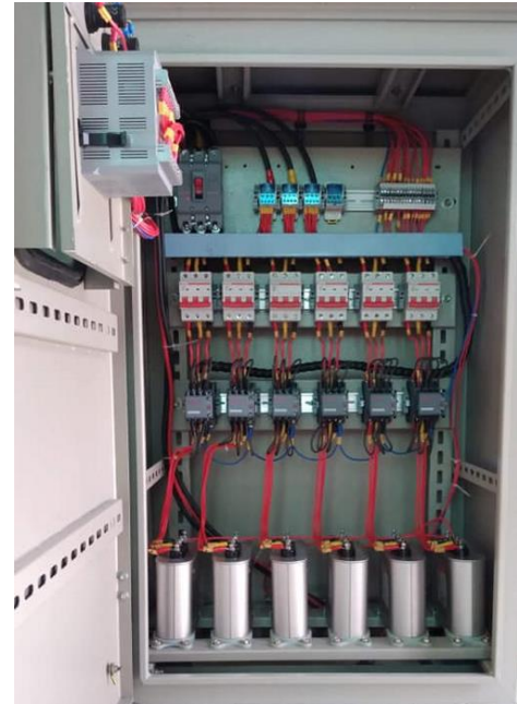
Fig 14. Capacitor Bank Control Panel
