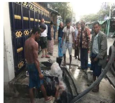
Fig 5.Physical losses due to leakage at cap
