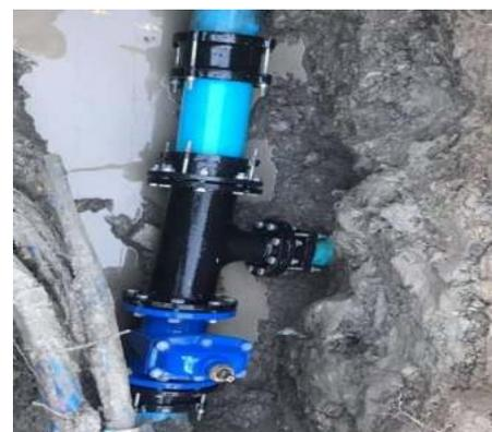
Fig 6.Physical losses due to joint error
